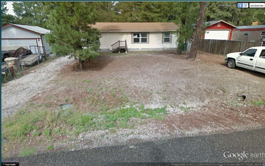
Figure 2: Residential Project Site
